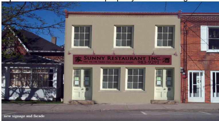
new signage and facade
